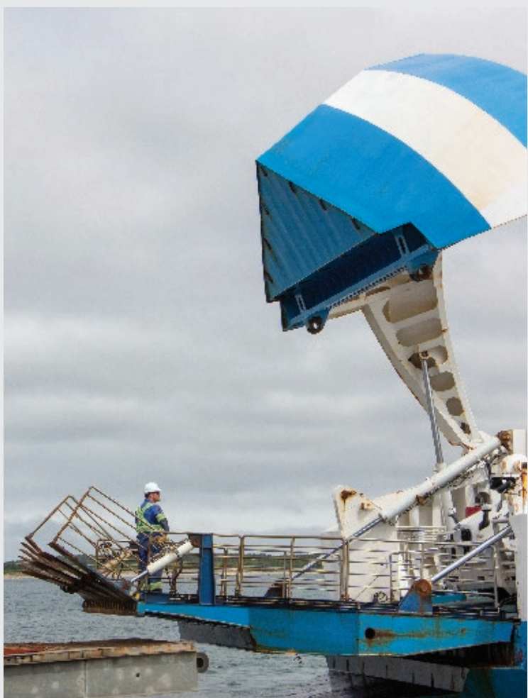
Qajak W. (Ferry Ramp).
